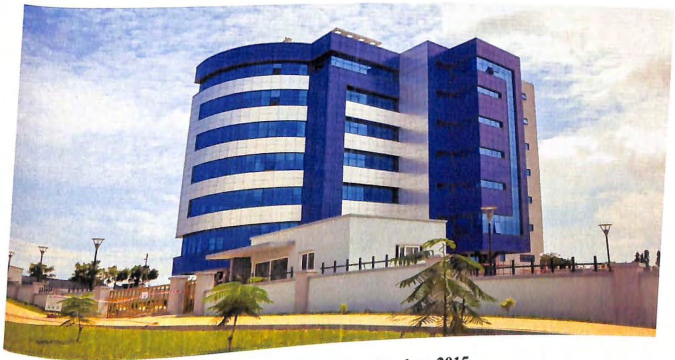
Figure 11: The New GATA Complex completed in October, 2015
