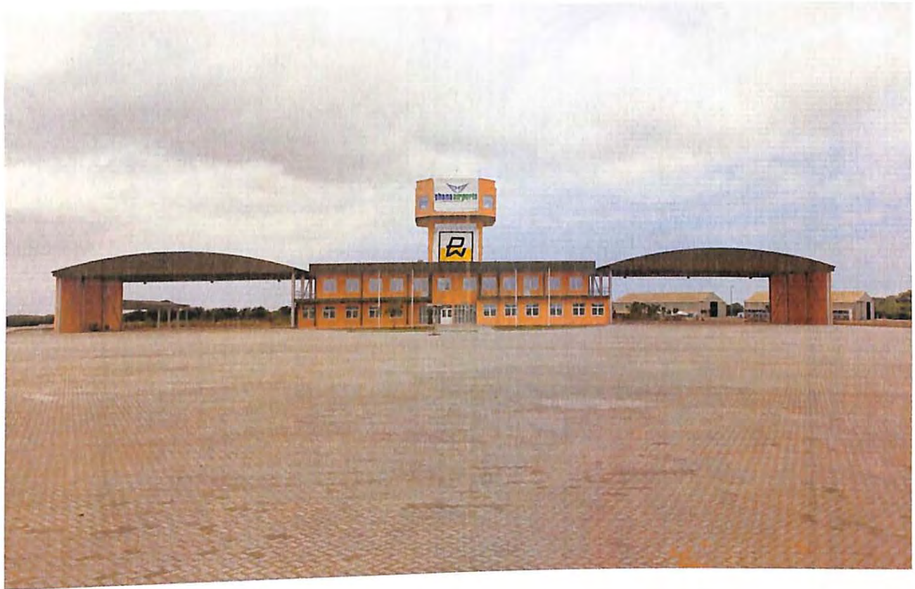
Figure 7 New Rescue & Fire Fighting Station
