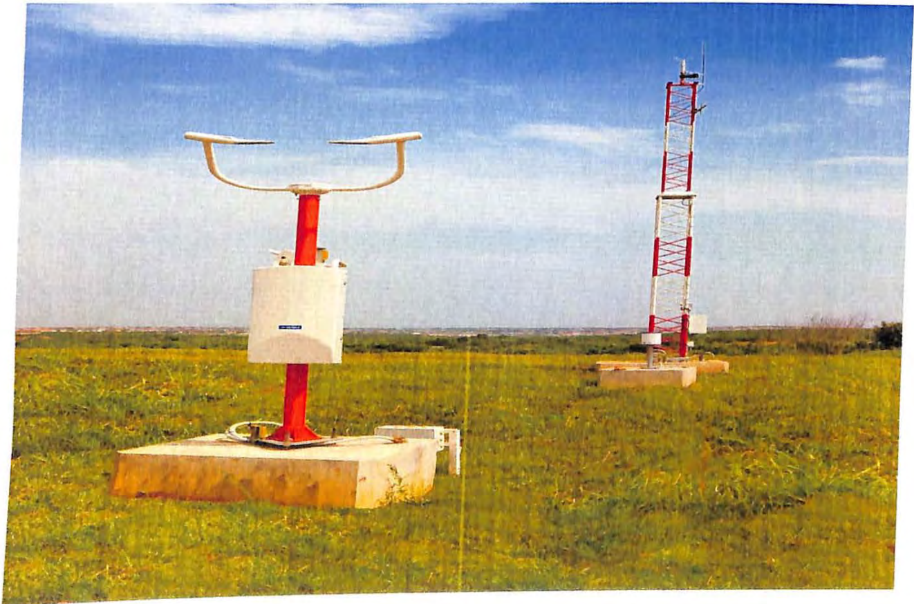
Figure 6(a): Automatic Weather Observation System
