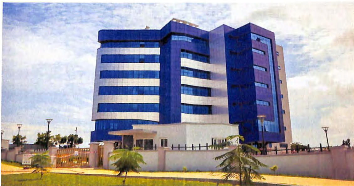
Figure 11: The New GATA Complex completed in October, 2015
