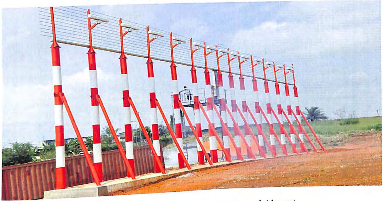
Figure 5(a): Instrument Landing System (ILS) at the Kumasi Airport
