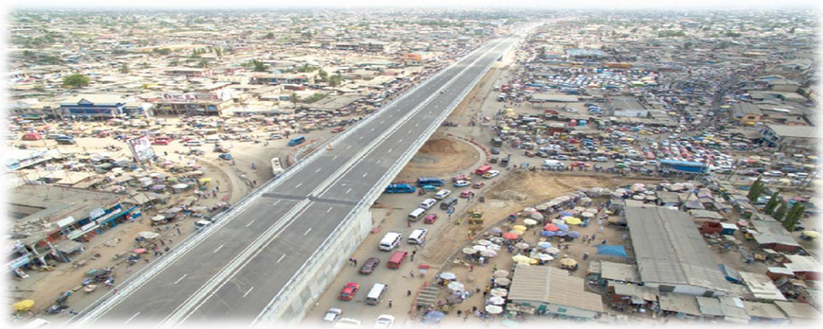
Figure 5: An Overview of Kasoa Township
